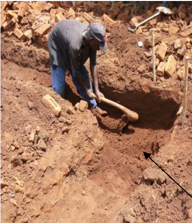
Excavation for Furnace Foundation
