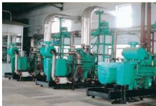
Figure 1. 100% producer gas engines at 1 MW power station in Tamil Nadu State (Source: MNES)
