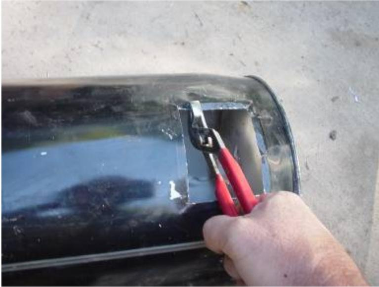
As before, use tin snips to cut out the rectangular area as marked. Then, fold the edge at the placement mark, and bend back the metal by striking with the ball-peen hammer.
